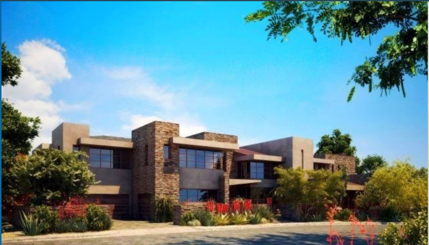
NAHB New American Home, Las Vegas. Exterior and interior walls insulated with cellulose for thermal efficiency, sound transmission control and fire safety.
