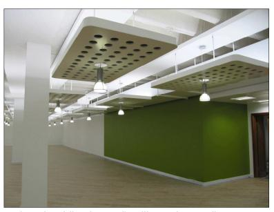
surfaces (such as water stained ceilings, wood and oxidized metal) will require sealing to prevent migratory staining of the SonaSpray finish. SonaSpray fc can be installed where panels or stretch fabrics are impossible and with thin coatings is the best sound absorber.
